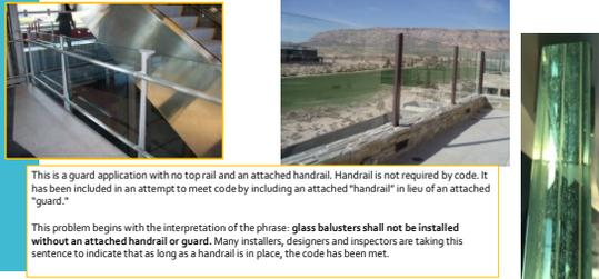
This is a guard application with no top rail and an attached handrail. Handrail is not required by code. It has been included in an attempt to meet code by including an attached "handrail" in lieu of an attached "guard."
